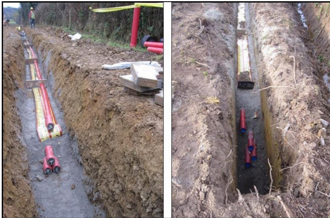
Figure 2.12 Typical Cable Trench (Extracted from CEMP)
