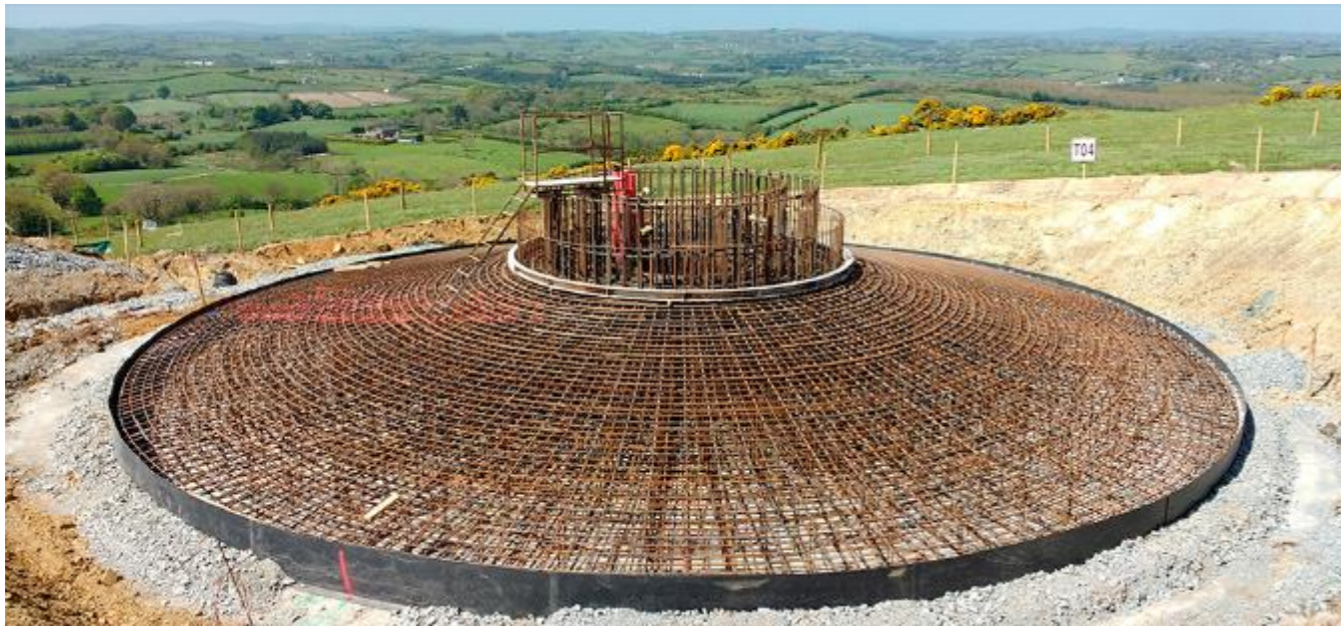
Figure 2.2 Sample Image of Turbine Foundation Anchor Cage
