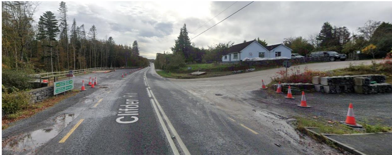
Figure 5.1 Improved N59 / L-53453 Junction - looking south along the N59 with layby / turning area on left (Source: Google Maps)
